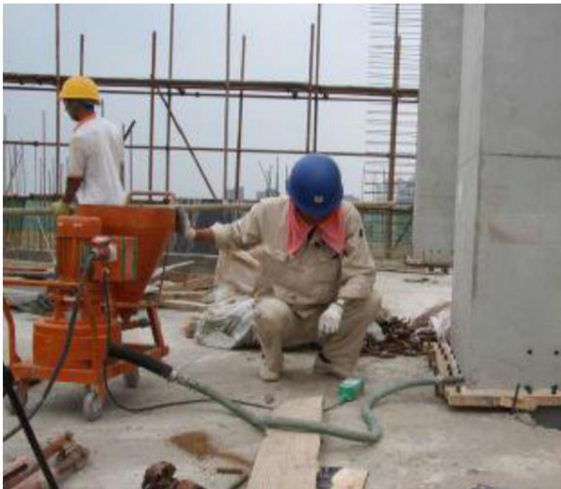
Mechanical grouting
