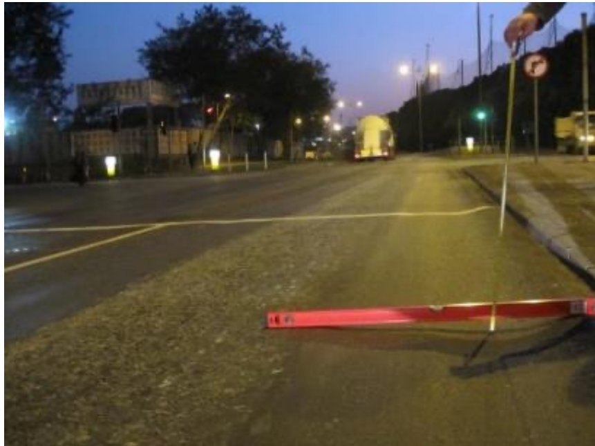
Pavement Rutting Due to Slow and Heavy Traffic
