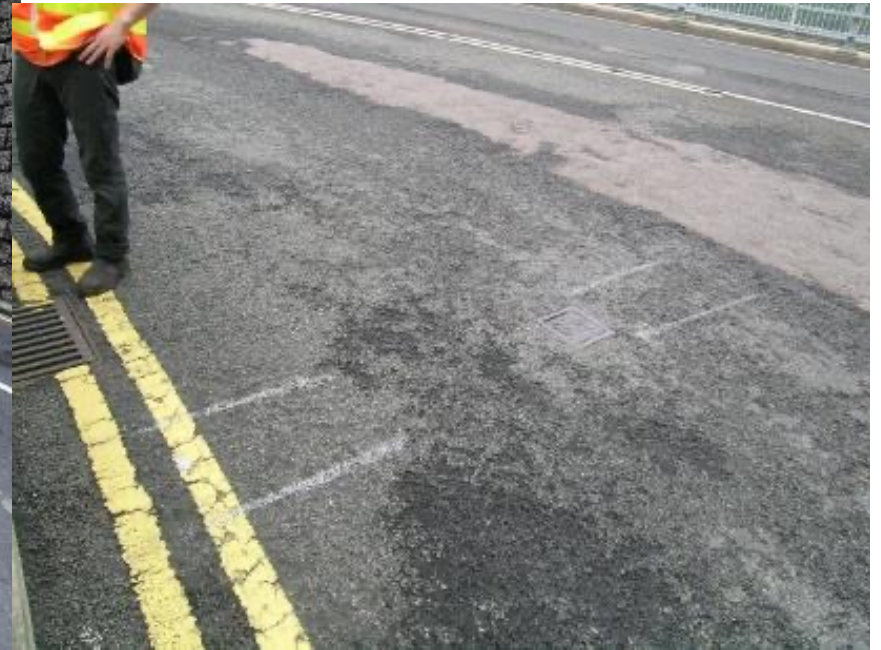
Raveling of Porous Pavement
