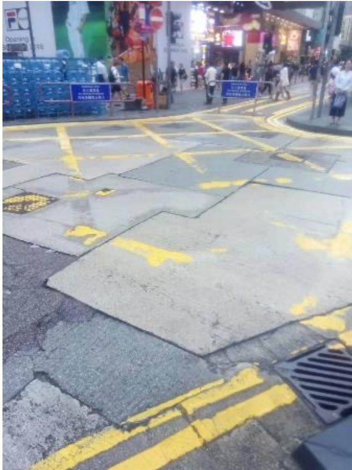
Pavements after “Quick” Repairs
