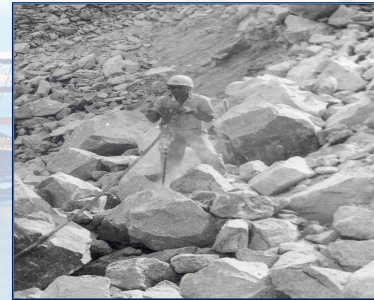
Drilling Techniques by manual hydraulic breaker without any PPE
