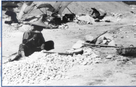
Grading of Rock into aggregates manually
