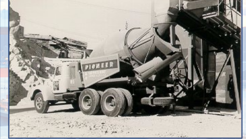
Concrete loading into the mixer truck in open area
