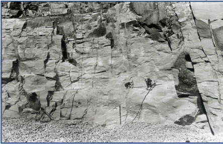
Powder Monkey's for installation of explosive without any safety measures
