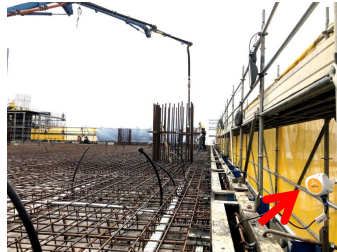
Install sensor before concreting
