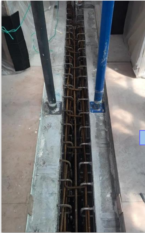
Casting by Self-Compacting Concrete
