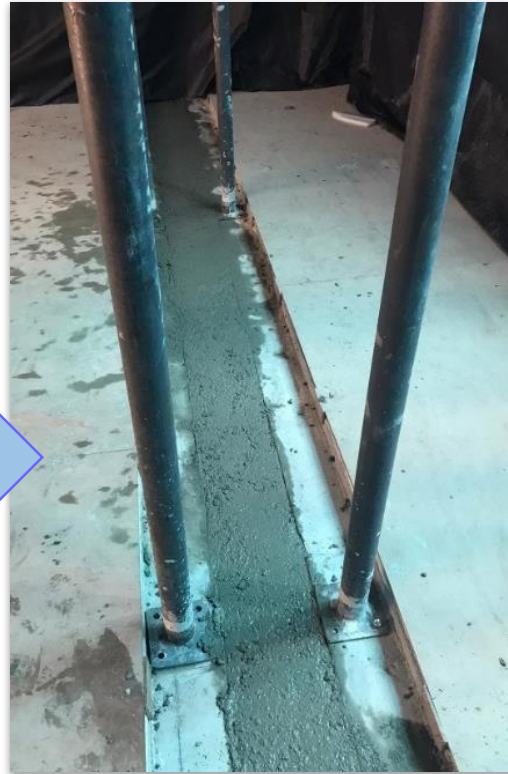
Casting by Self-Compacting Concrete
